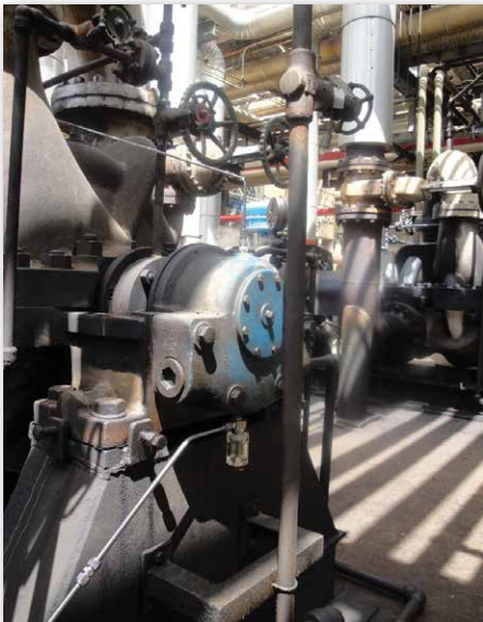
Figure 1: Pure oil mist in centrifugal pump. Note the collecting bottle at bottom of pump bearing housing.
